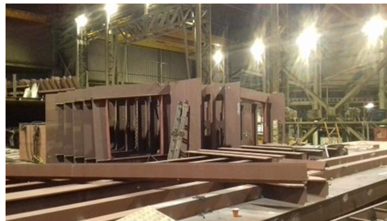
Block construction September 2020
